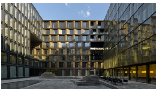
Europaallee 21, Construction Area C, Zurich, CH
