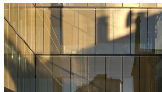
C Quadro, Executive Building, Udine, IT
